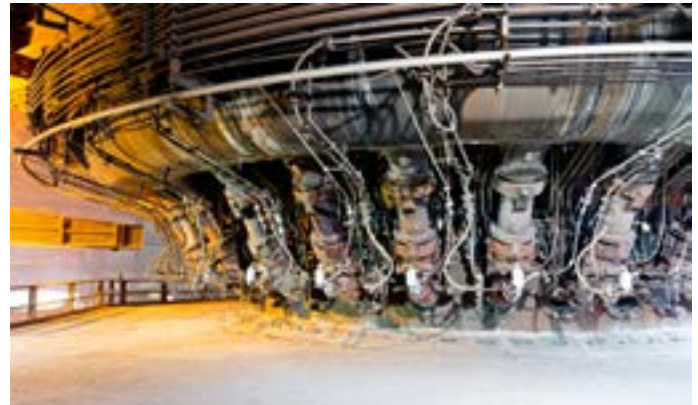
Tuyeres Mounted Around Blast Furnace
